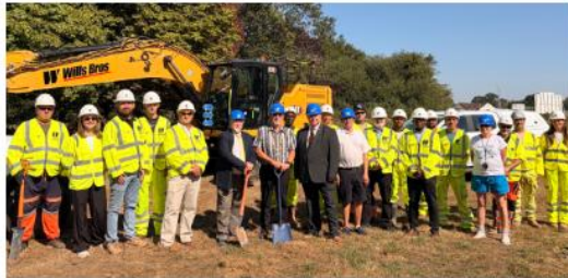
Members of construction team Wills Bros with Cllr Steve Keable, Cllr Tony Spring, Cllr James Buczkowski, for the three councils involved.
