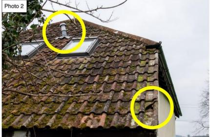
Several tiles along the southern edge of the roof have been cracked (see photo 2) and last week we replaced nine cracked tiles on the eastern edge of the roof. Photo 3 shows a particularly badly damaged tile before it was replaced. Tiles on the roof of our woodshed have also been damaged, presumably also by footballs which are frequently kicked over the Stables and land in our garden and driveway.
